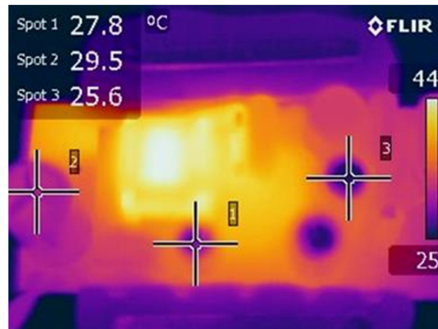
Figure 24 – SP1 – Bias Capacitor (C5). SP2 – Output Capacitor (C11). SP3 – Valley Fill PFC Capacitor (C1).
