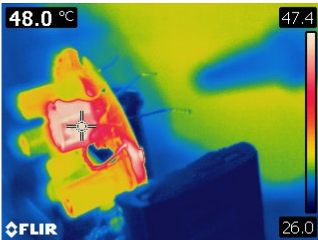
Figure 35 – 265 VAC 50 Hz, Full Load. Power Transformer (T1): 48.0 °C.
