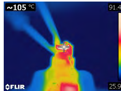
Figure 22 – Fusible Resistor (R1) = 105 °C.
