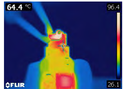
Figure 23 – Damper (R10) = 64.4 °C.
