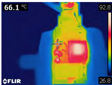
Figure 33 – Damper (R2) = 66.1 °C.
