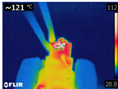
Figure 40 – Fusible Resistor (R1) = 121 °C.
