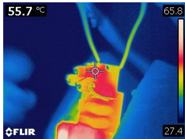
Figure 21 – 120 VAC, 72 V LED LOAD. Spot 1: Fusible Resistor (RF1): 55.7 °C.
