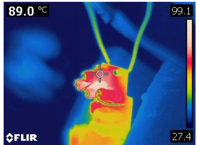
Figure 25 – 120 VAC, 72 V LED LOAD Spot 1: Fusible Resistor (RF1): 89 °C.
