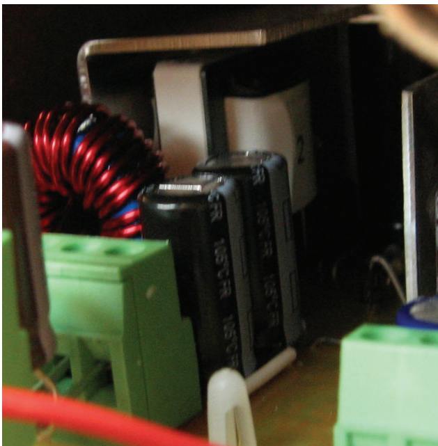
Figure 60 – Main Output Transformer T1, Visible Light View.
