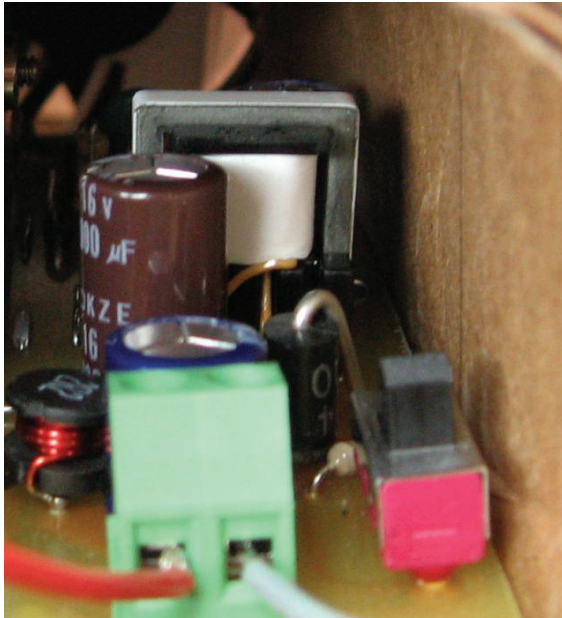
Figure 54 – Standby Transformer T2, Visible Light View.
