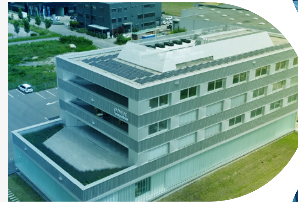
25 kW system at our Biel, Switzerland, facility
